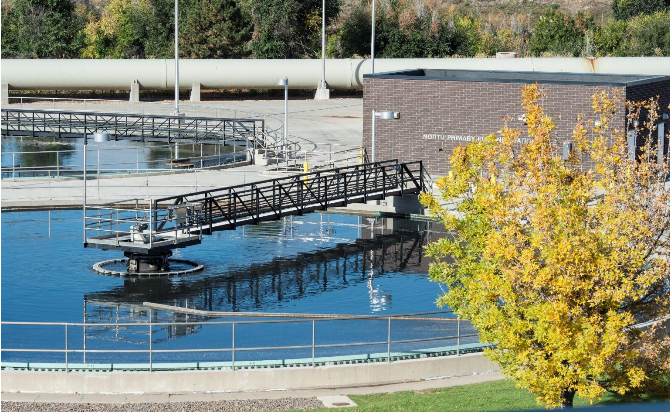
Robert W. Hite Treatment Facility in Autumn.
